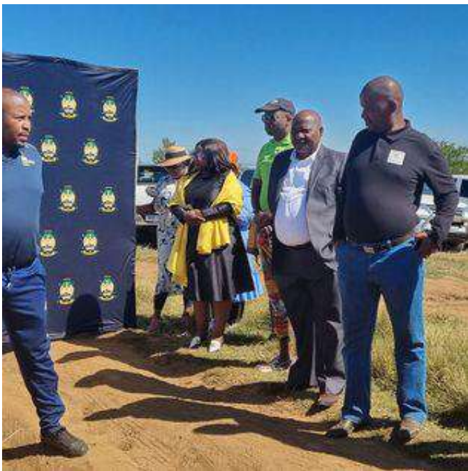
Picture 5: Site and Contractor Handover of Echibhini Access Road , in the picture we have Mayor: Cllr NW Ntombela, Speaker : Cllr TA Gwala, Deputy Mayor: Cllr Maphanga , Inkosi Maphumulo from Mbambangalo TC along with the contractor.
