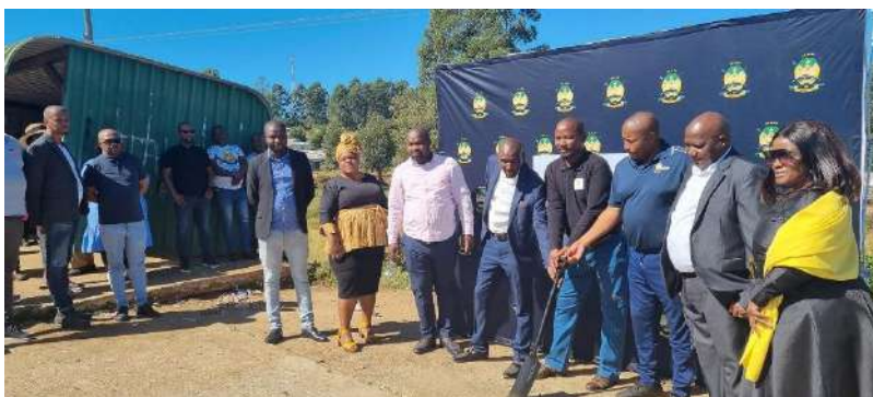
Picture 3: Site and Contractor Handover for Maqongqo Taxi Rank in the picture we have Mbamabangalo TC : Inkosi Maphumulo , Cllr Maphumulo who is the Ward 1 councillor and Mayor : Cllr NW Ntombela holding the spade of site for Maqongqo Taxi Rank.
